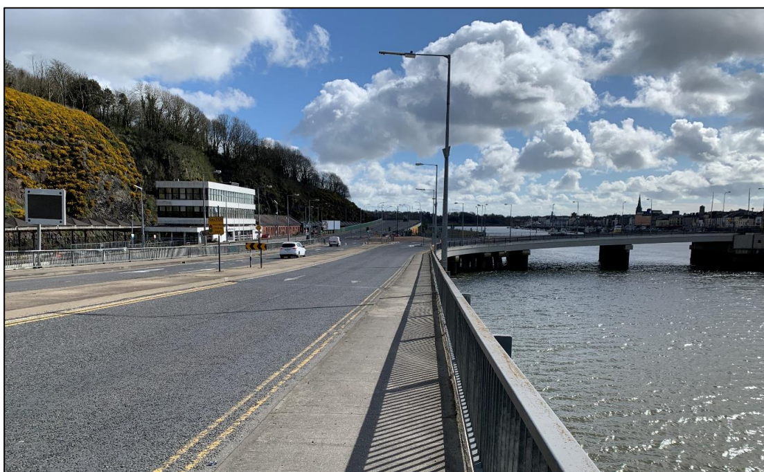
Plate 11.3 View east along Terminus Street with rockface / ridgeline to left (north) and River Suir (south); note that rail below is screened from angle of view from elevated road.
