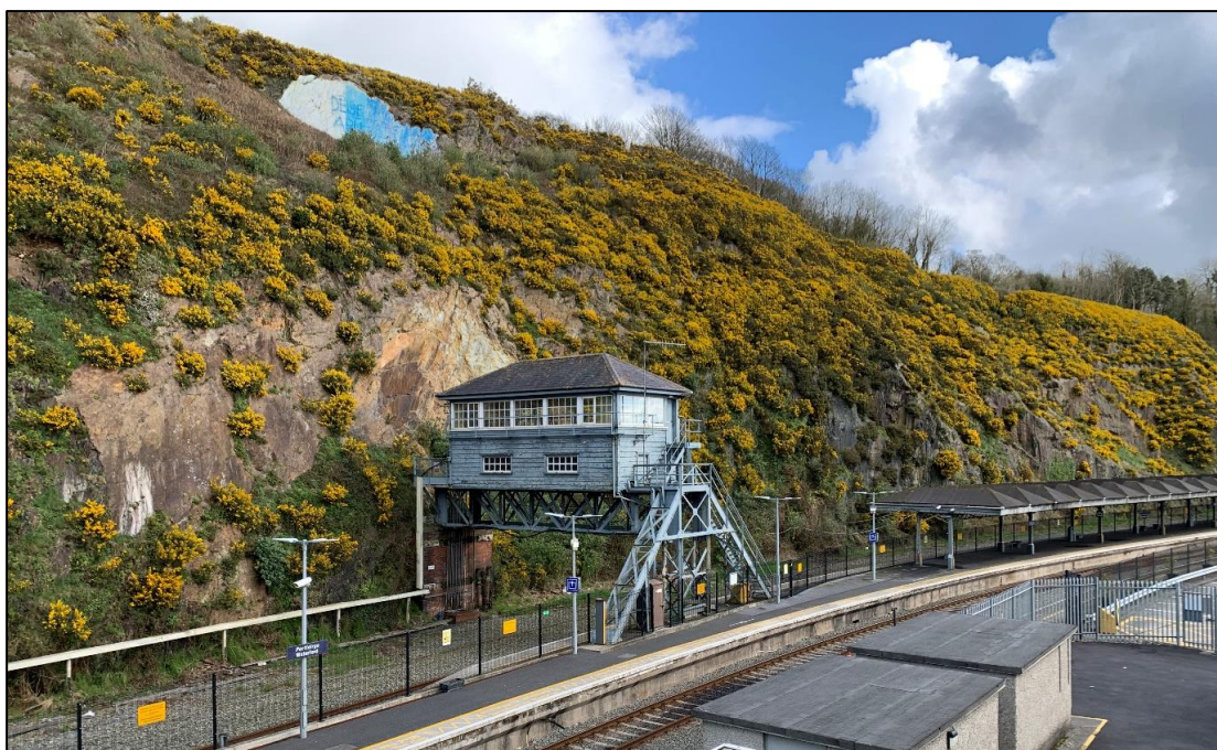
Plate 11.5 19 th Century Signal Tower, west of Plunkett Station (listed building) with rock face behind
