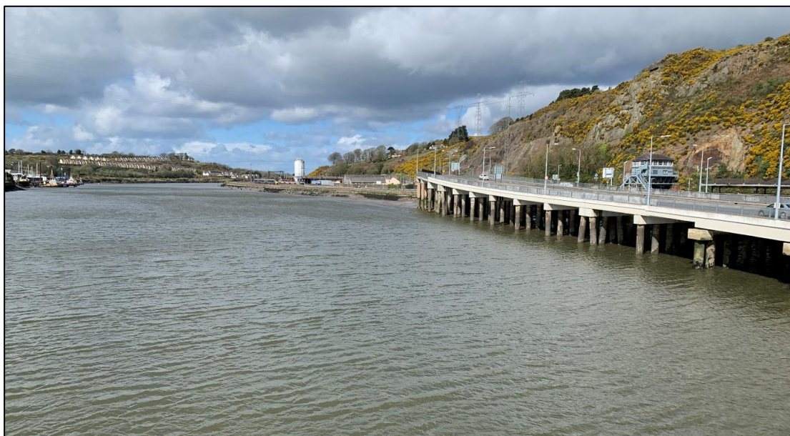
Plate 11.9 Rice Bridge looking west – views from footpaths
